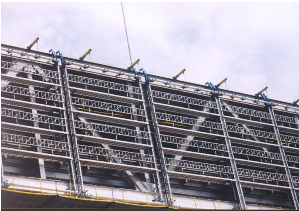
Cable Supported Platform/Scaffold
