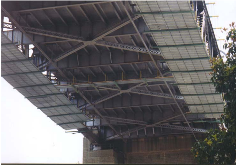
Lower Truss Chord Platforms
