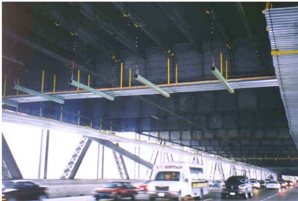
View Showing Cross Over Platforms
