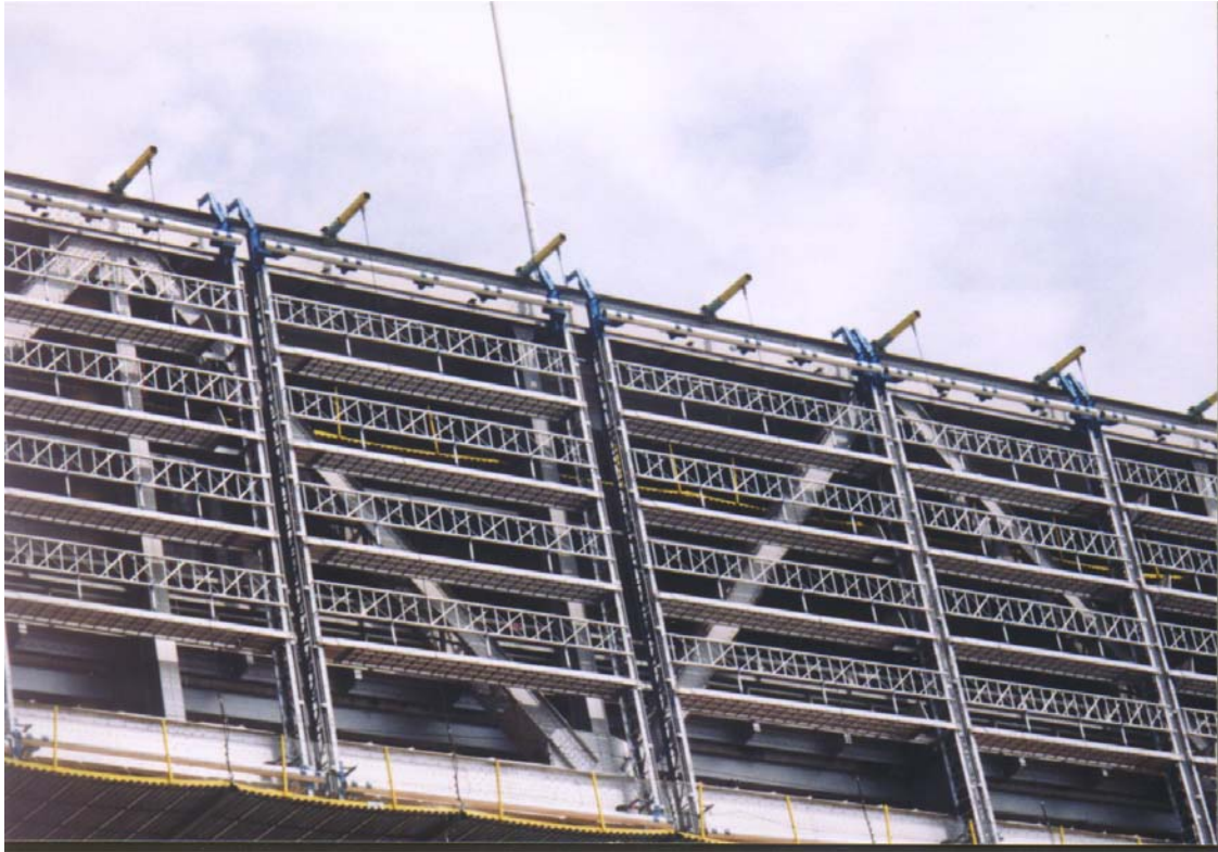
Lower Truss Chord Platforms Scaffolding
