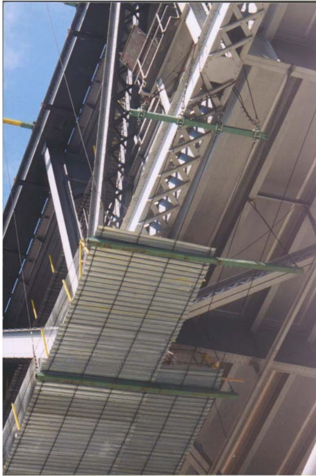
Platform Below Lower Truss Chord
