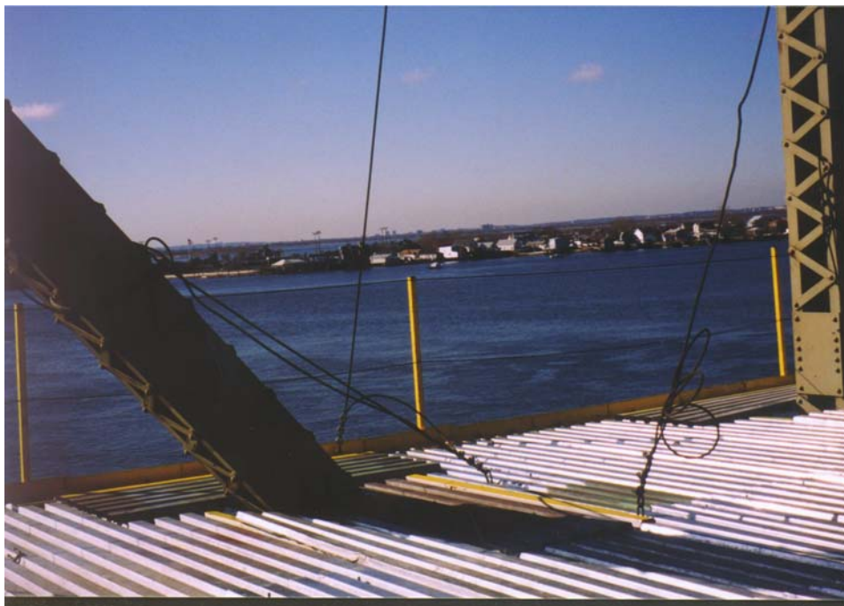
Intermediate Cable Supported Platform
