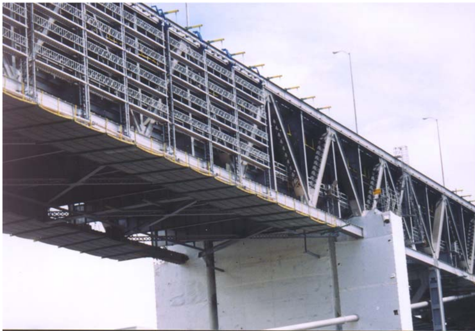
Platforms Below Lower Truss Chords
