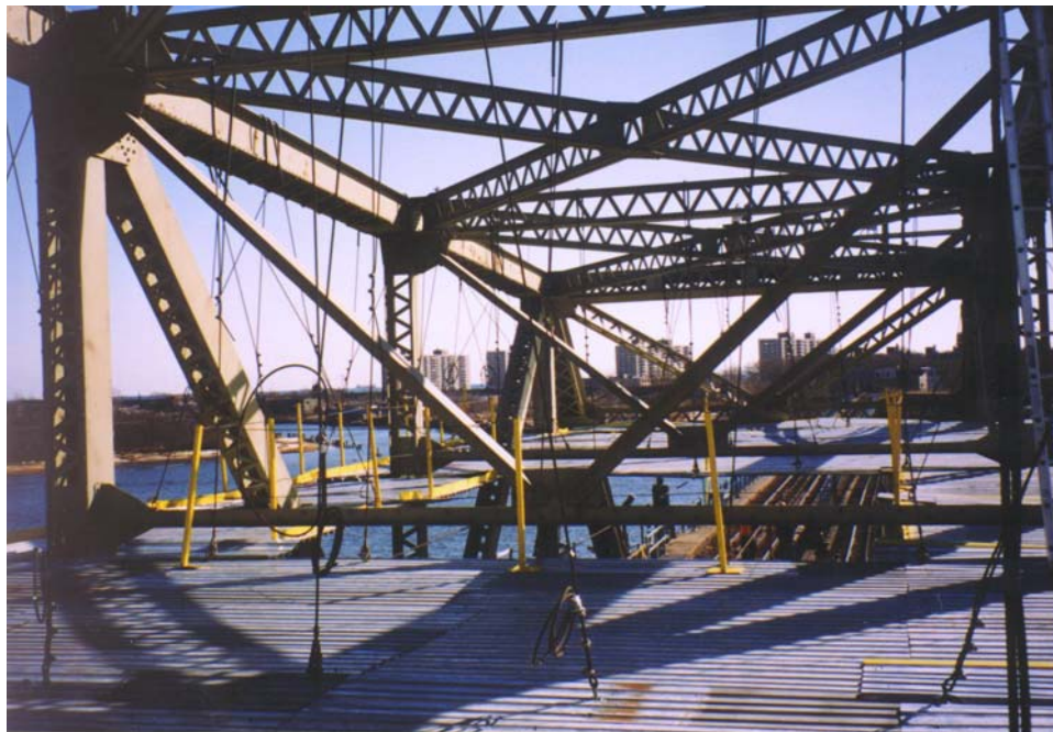
Intermediate Level Cable Supported Platform
