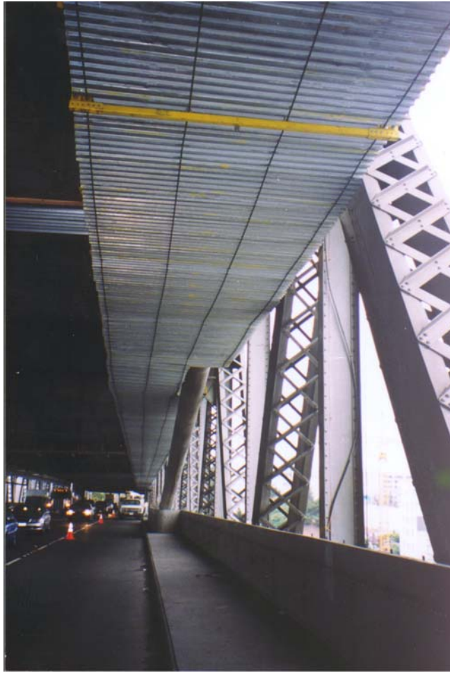
Cable Supported Platform
