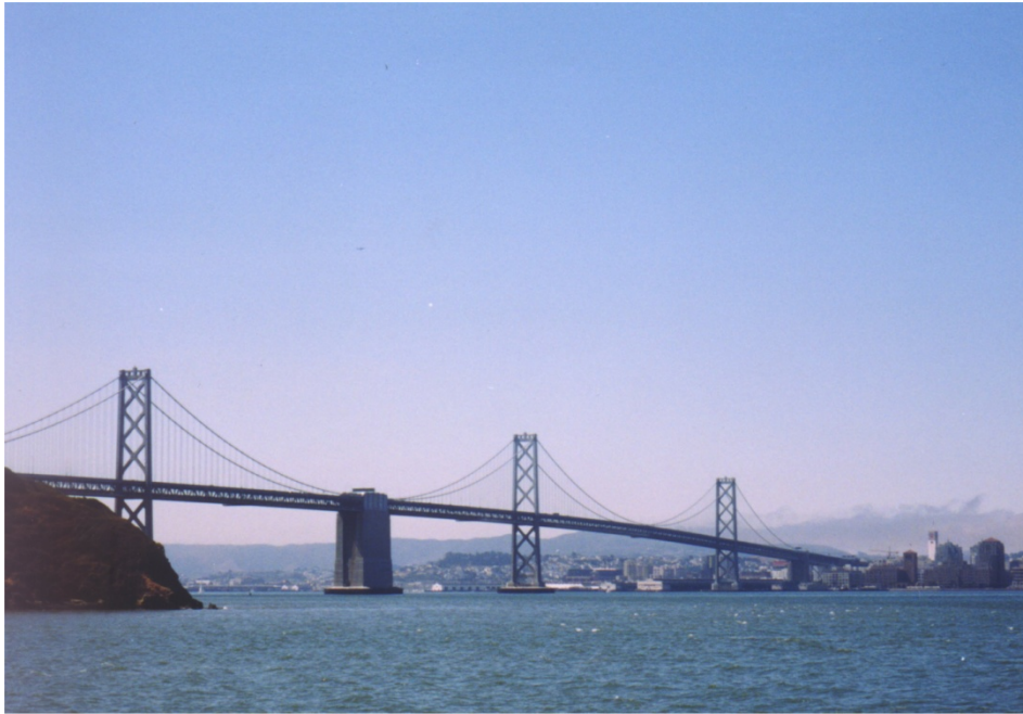
Cable Supported Platform
