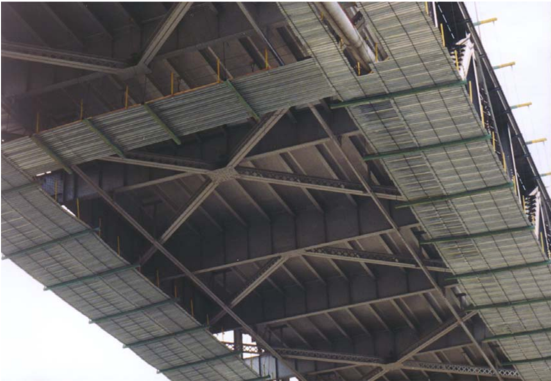
Lower Truss Chord Platforms & Crossover
