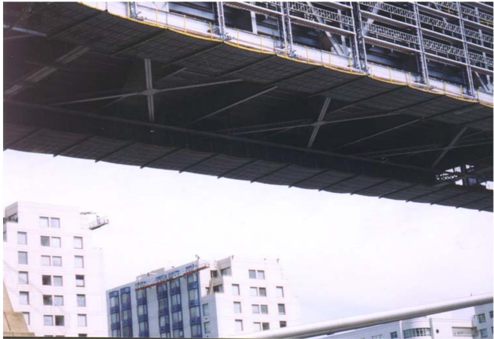
Platforms Below Lower Truss Chords
