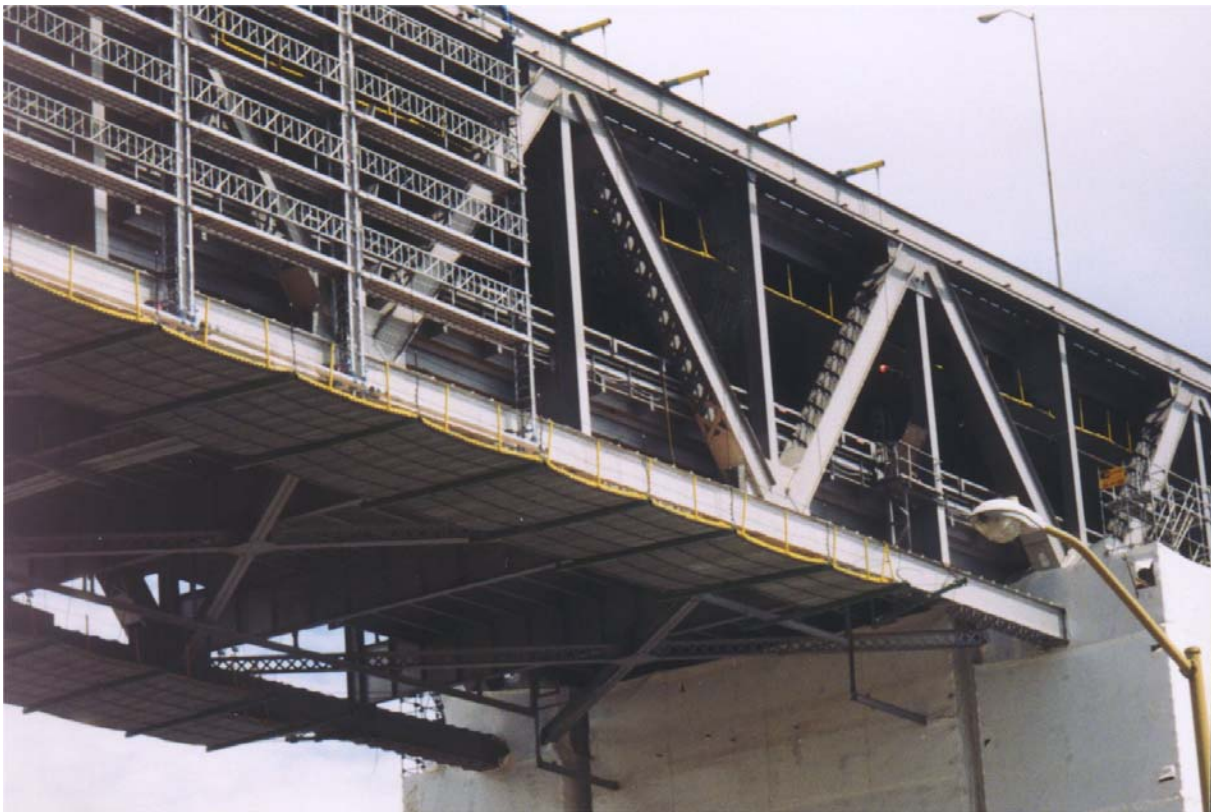
Lower Truss Chord Platforms Scaffolding
