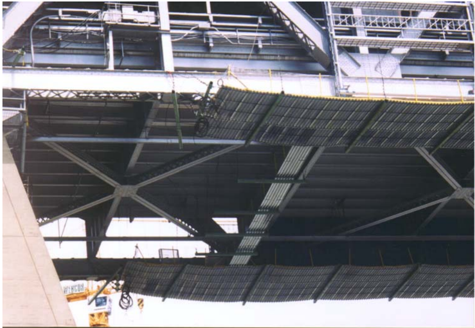
Platforms Below Lower Truss Chords & End Connection
