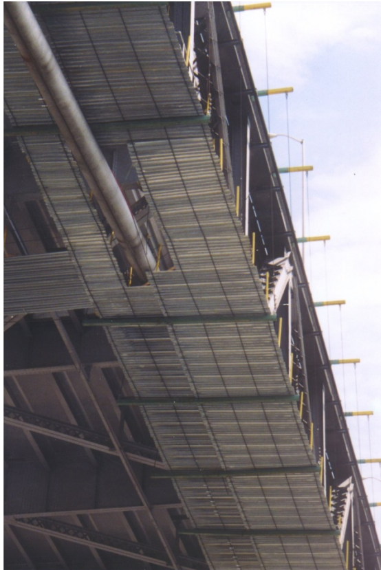
Platform Below Lower Truss Chord
