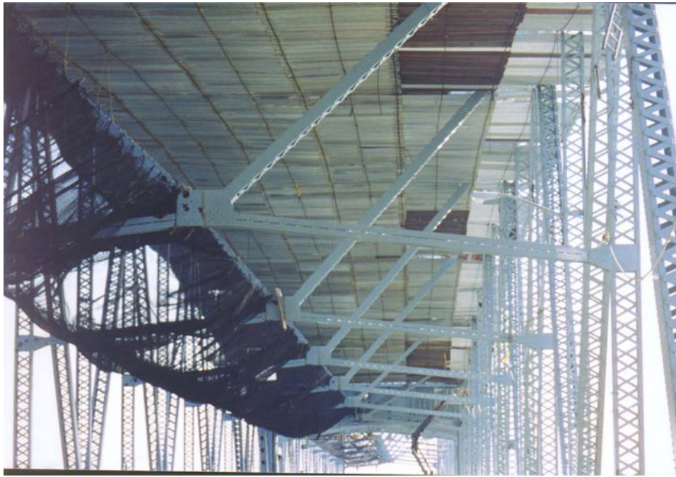
Upper Level Platform & Debris Netting
